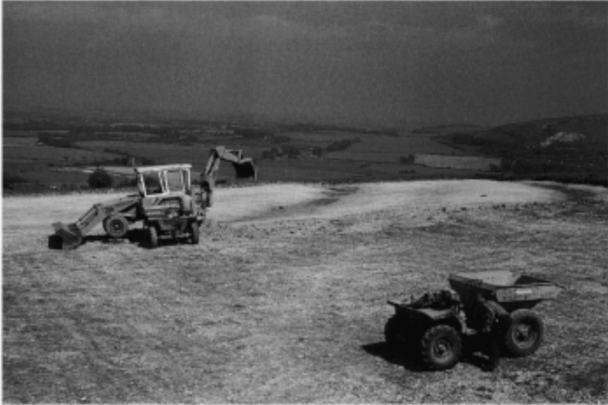
Figure 5.13 Coarse excavation: digging with a JCB 3c.
