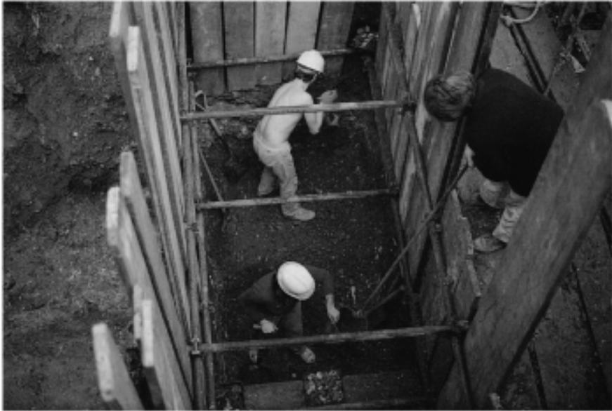
Figure 5.2 Site safety: shoring of a narrow trench.
