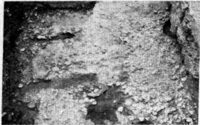
Fig 16 Peter's Hill; first chalk raft showing an uneven (nodular) and uncompacted finish outside the line of the later foundation. (Scale 10 x 0.10m)
