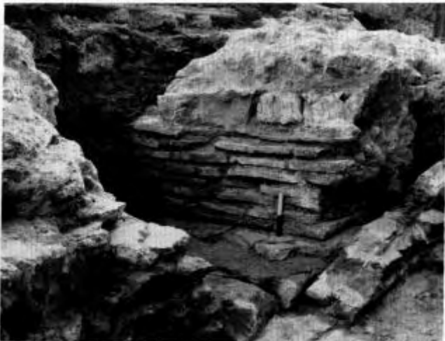
Fig 22 Sunlight Wharf; culvert within the monumental foundation (looking south-west). The base of the culvert utilised the re-used blocks of the monumental foundation. The sides were tile built for the first 0.3m, and then the core of the monumental foundation was faced with ragstone. (Scale 2 x 0.10m)
