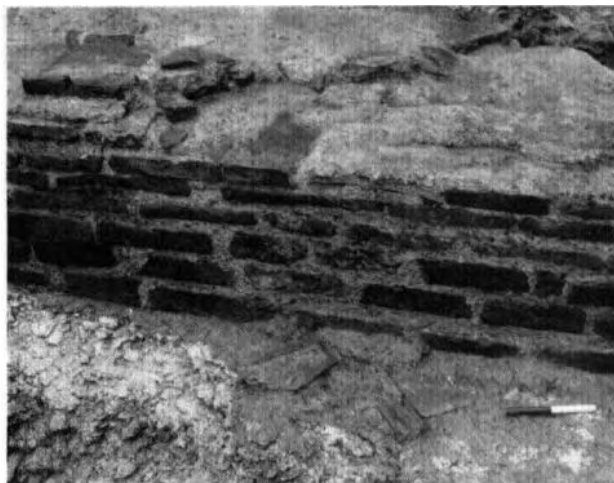
Fig 45 Peter's Hill; detail of the tile built terrace wall, showing construction debris in the foreground. (Scale 2 x 0.10m)
