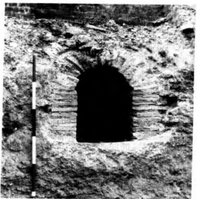
Fig 60 Culvert piercing the long wall at Knightrider Street (Observation 16). (Scale 6 x 1')
