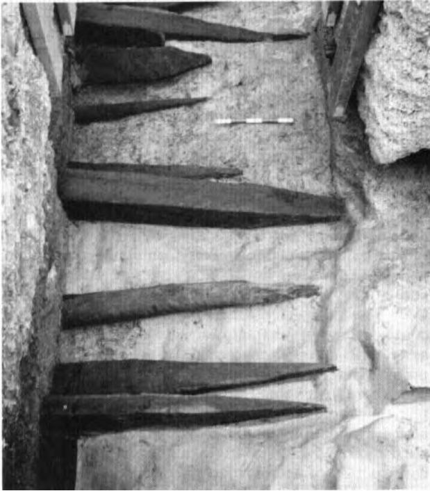
(a) layer of sharpened timbers, laid on the natural clay.
